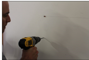
(11) Remove unit and drill holes for lower two positions.
