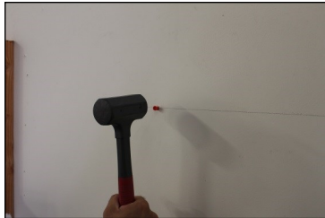
(7) Tap wall anchors into both holes.
