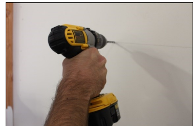
(6) Drill 3/16" holes in the two marked positions.
