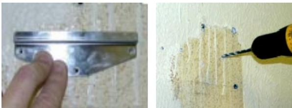
(3) Press in the dry wall anchors and mount the bracket.
